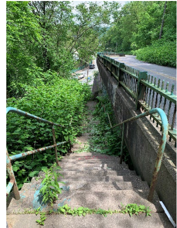
Steps at Baker Street and Butler Street
