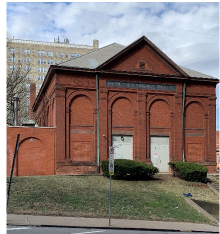
Herron Hill Pumping Station
