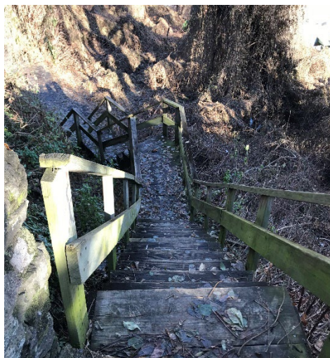
Former Mackey Street Steps Viewed from Lawn Street
