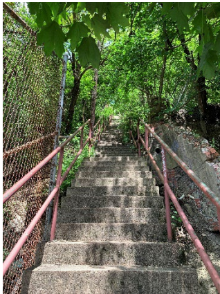
Vinial Street Steps
