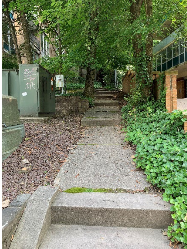
Devon Road Steps
