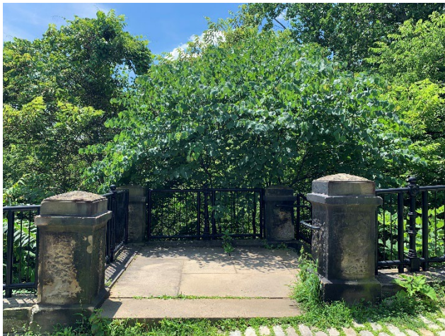
Entrance to First Set of Lower Panther Hollow Trail Steps
